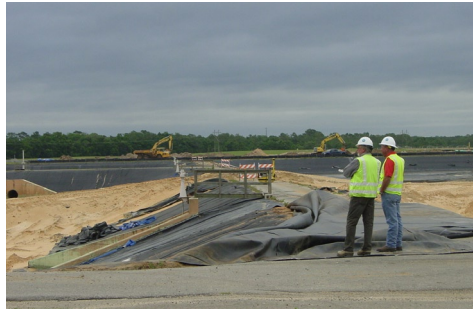
Crew look over the site where work has begun on the Advanced Wastewater Treatment facility.
