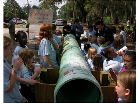
The group gathers around to sign the pipe before it is placed into the ground on Gaines Street.
