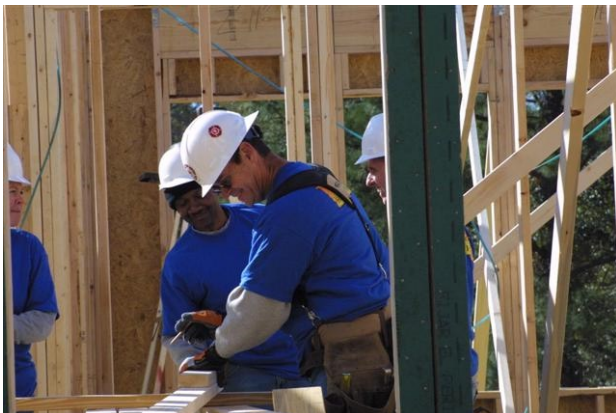
Firefighters volunteer their expertise during the EMHE build.
